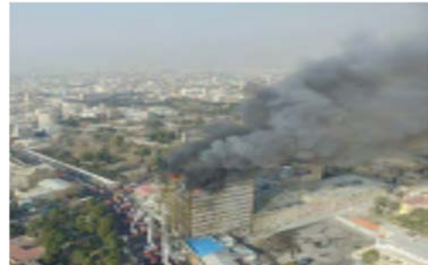
Figure 3: Aerial view of the building during the fire on January 19, 2017, showing the shopping mall at rear.
